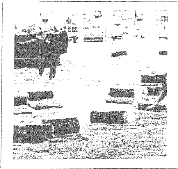
Exhibit 3.14-C. Lay the strips of sod in a staggered, brick-like fashion.
