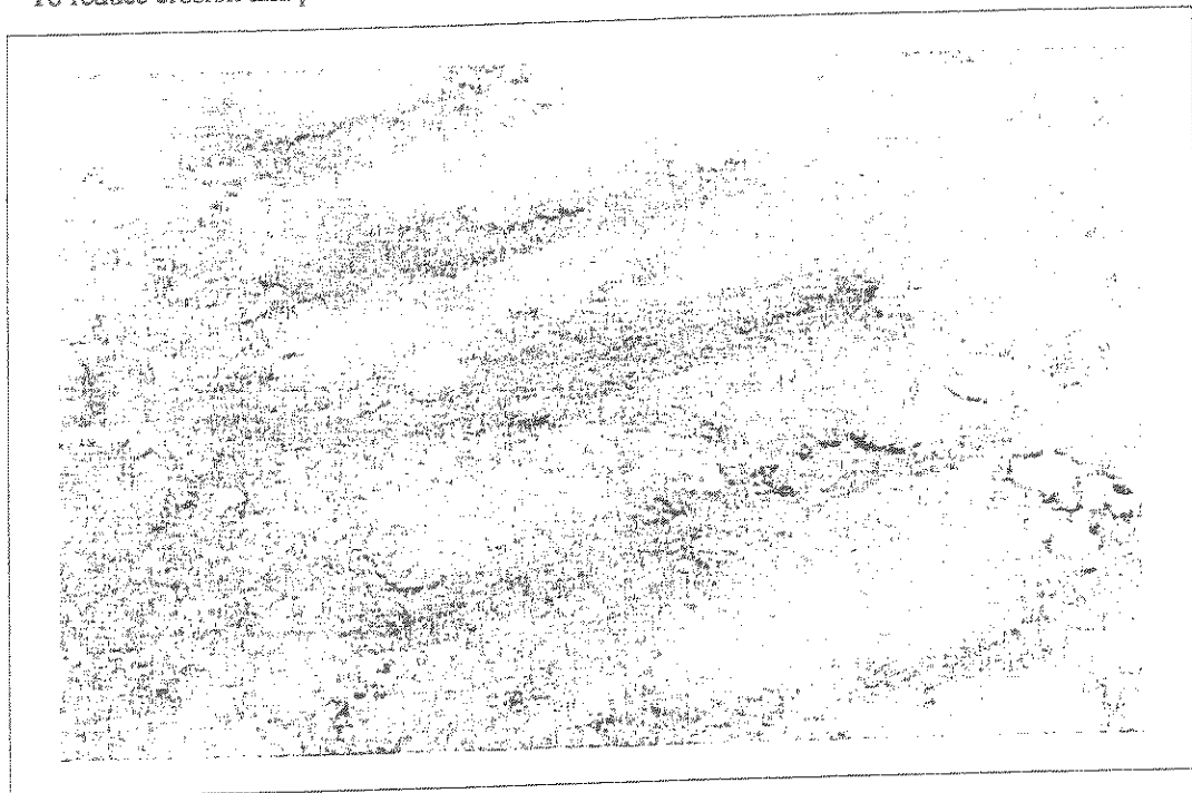
Exhibit 3.03-A. Surface roughening by bulldozer cleats.
