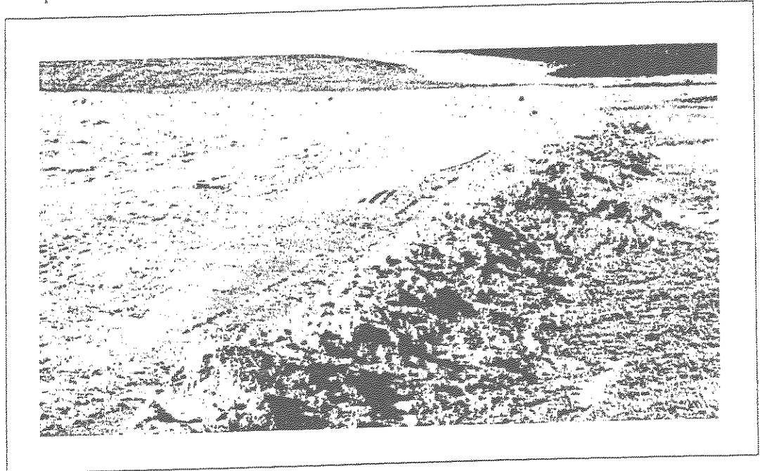
Exhibit 3.21-A. A temporary earthen diversion.
