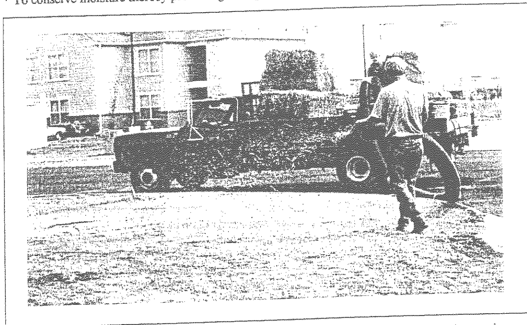
Exhibit 3.15-A. Applying straw mulch with a chopper-blower on freshly seeded soil adjacent to a road.
